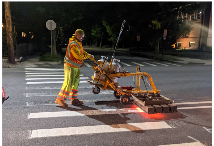
Contractor installing fresh crosswalks
