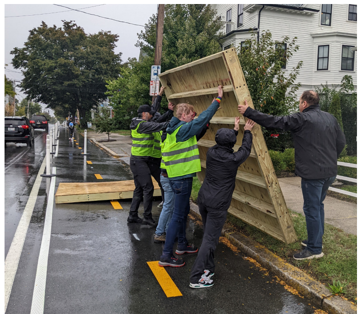
Volunteers installing the bus island in the temporary trail
